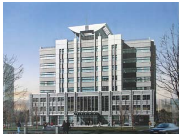
China's First LEED-Certified Building (Gold): National Research Center for Science and Technology for Development.
