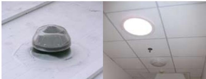
Rooftop collector for daylighting conduction device
