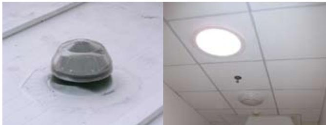
Rooftop collector for daylighting conduction device
