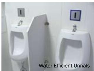
BEEC replaced inefficient water fixtures with newer, more efficient ones, additionally installing waterless and water efficient urinals, which when combined, save 28 percent more water than required by China's baseline water savings code.
