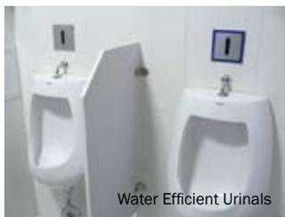
BEEC replaced inefficient water fixtures with newer, more efficient ones, additionally installing waterless and water efficient urinals, which when combined, save 28 percent more water than required by China's baseline water savings code.
