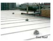
under the roof by 30 °C, lowering the building's indoor air cooling load in the summer. The cool roof also helps the building offset over 30 tons of carbon dioxide into the atmosphere every year.<sup>3</sup>
