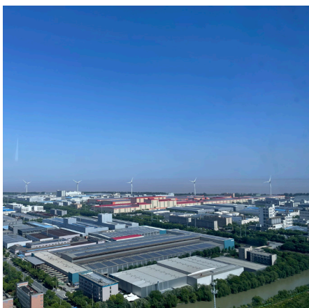
The rooftop solar and wind power in a Jiaxing industry park
